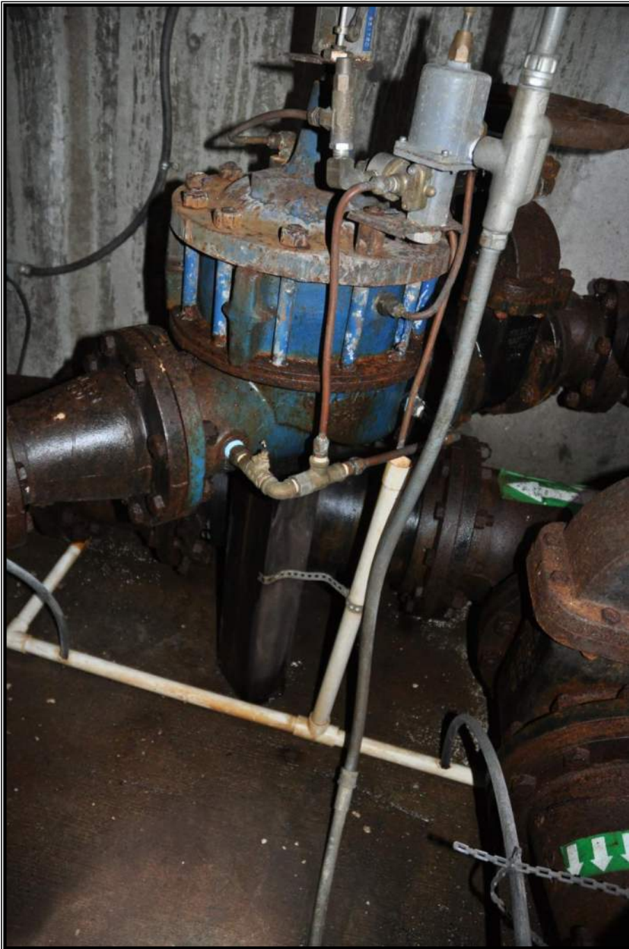
Martinazzi Pump Station – Outdated Pipe Bracing
