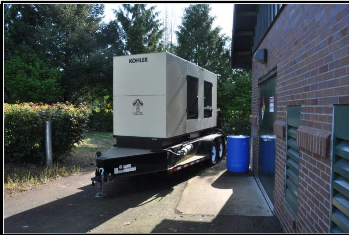
ASR Pump Station – Temporary Generator
