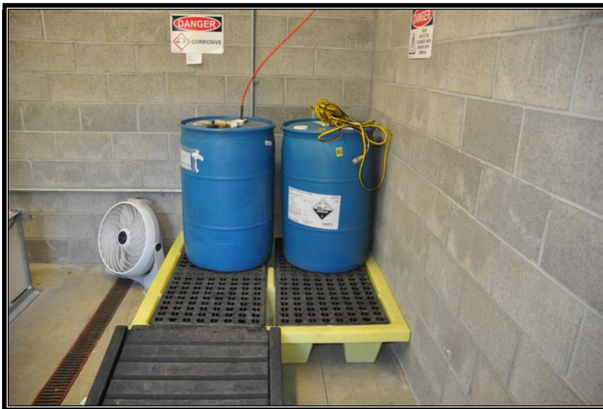
ASR Pump Station – Unbraced Chemical Barrels
