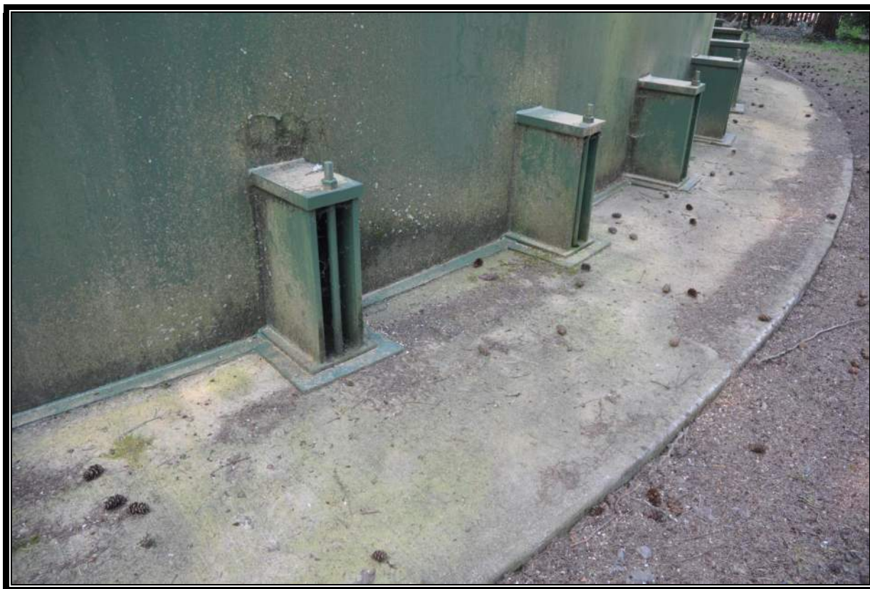
2.2 MG A1 Reservoir – Foundation and Anchorage Retrofit
