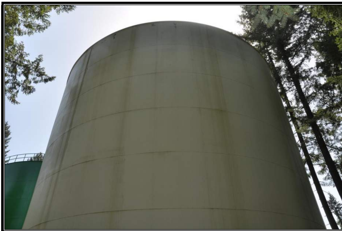
0.8 MG C1 Reservoir – Wall Shell Plates
