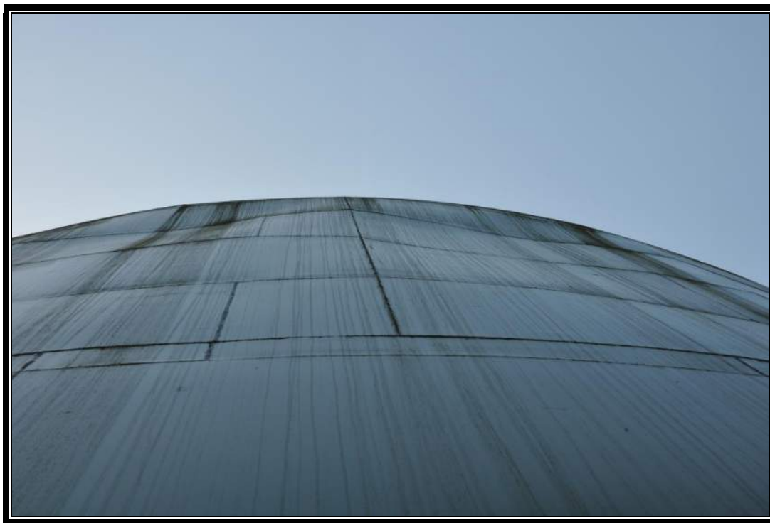
2.2 MG B1 Reservoir – Wall Shell Plate Buckling
