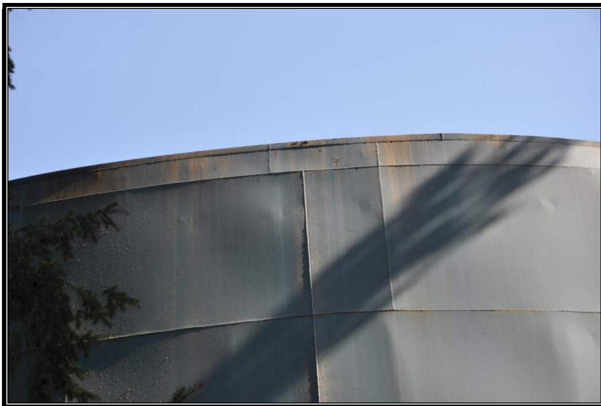
2.2 MG A1 Reservoir – Buckled Wall Shell Plates
