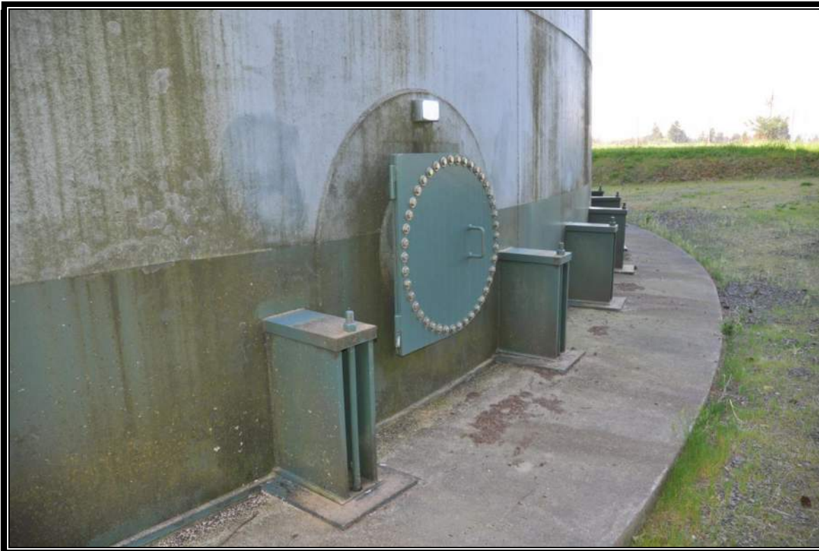
2.2 MG B2 Reservoir – Anchorage Retrofit
