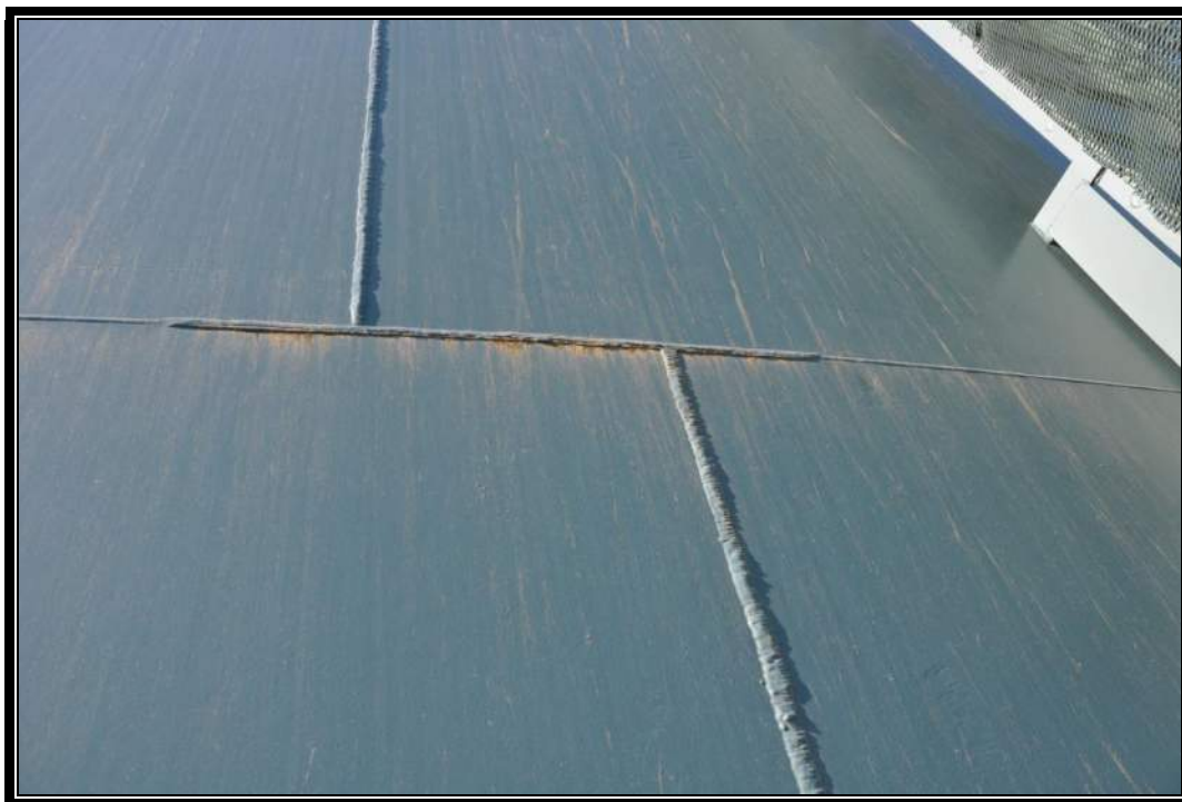
5.0 MG A2 Reservoir – Wall Shell Welds
