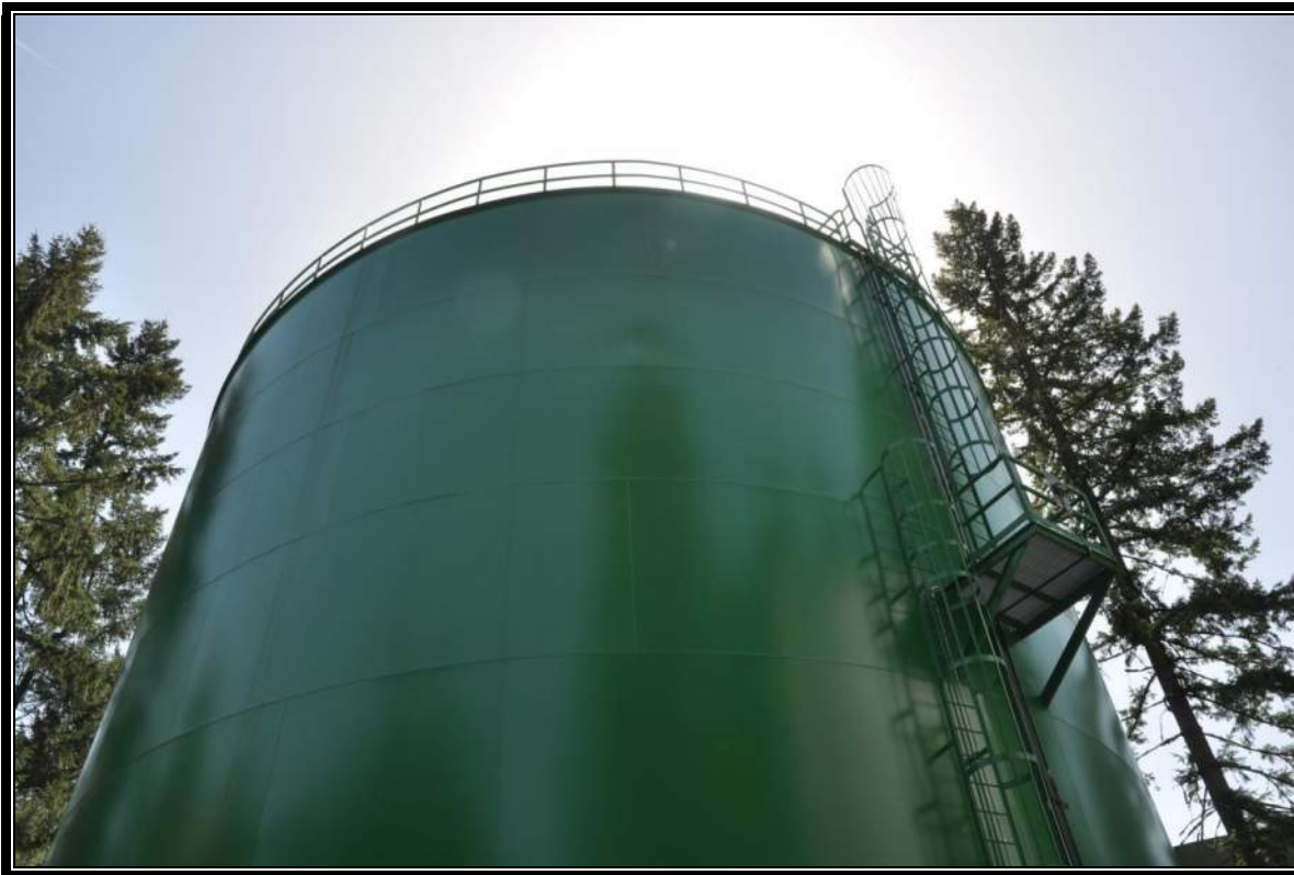
1.0 MG C2 Reservoir – Wall Shell Plates
