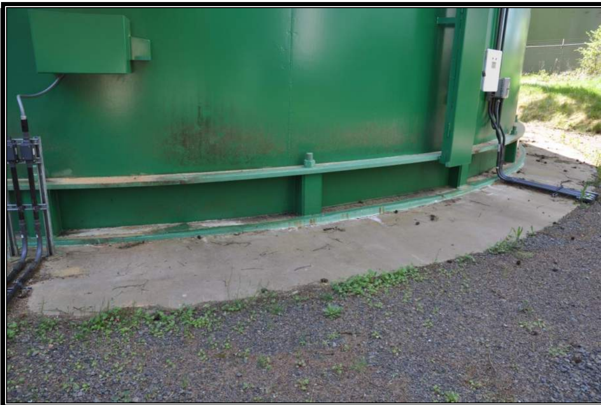
1.0 MG C2 Reservoir – Anchors and Foundation
