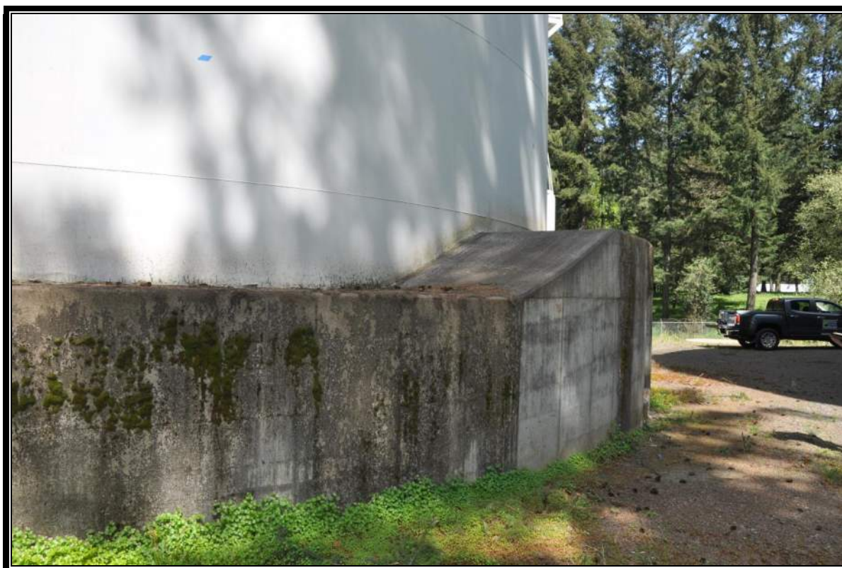
0.8 MG C1 Reservoir – Ballast Ring
