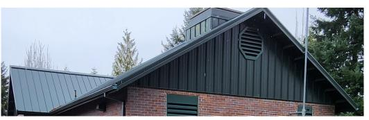
FOREST GREEN METAL STANDING SEAM ROOF, GUTTERS, AND DOWNSPOUTS TO MATCH EXISTING ASR BUILDING ROOFING
