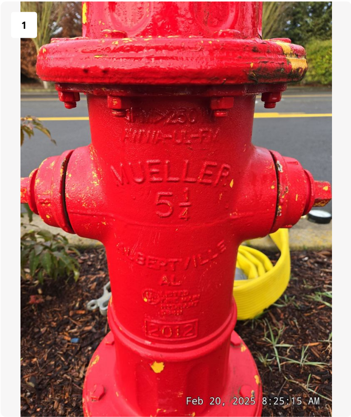
The flow hydrant, a Mueller 5 1/4.
