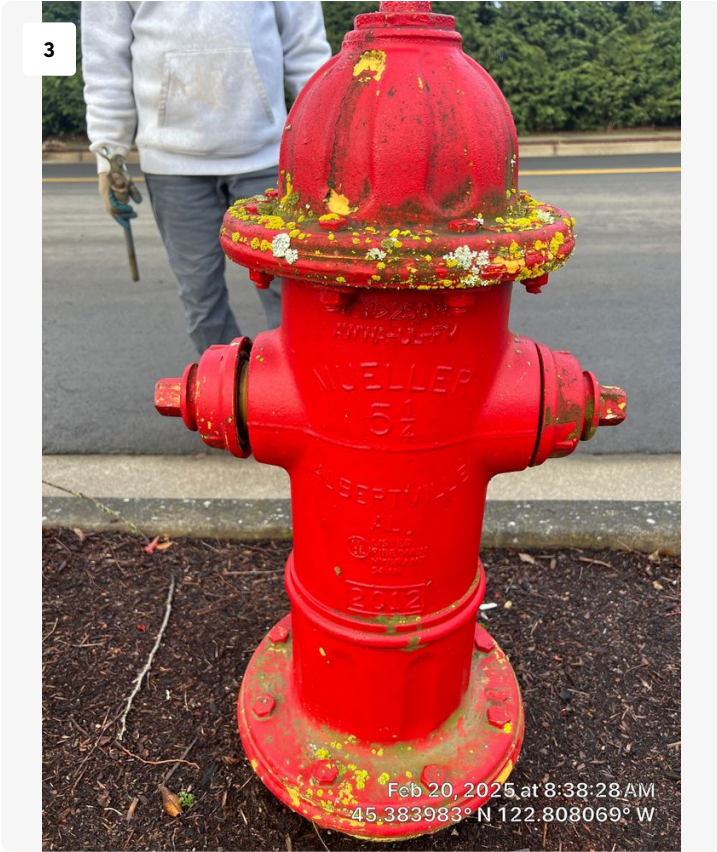
The gauge/residual hydrant, a Mueller 5 1/4.
