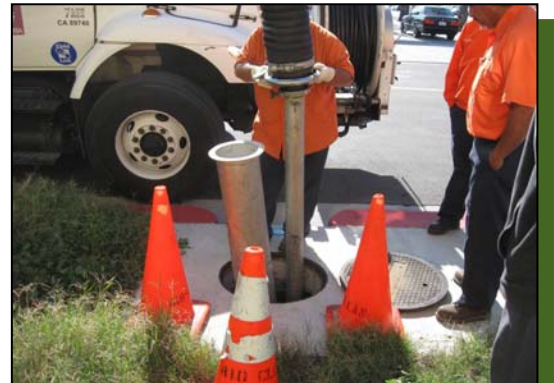
Insertion of vacuum hose into separation chamber.
