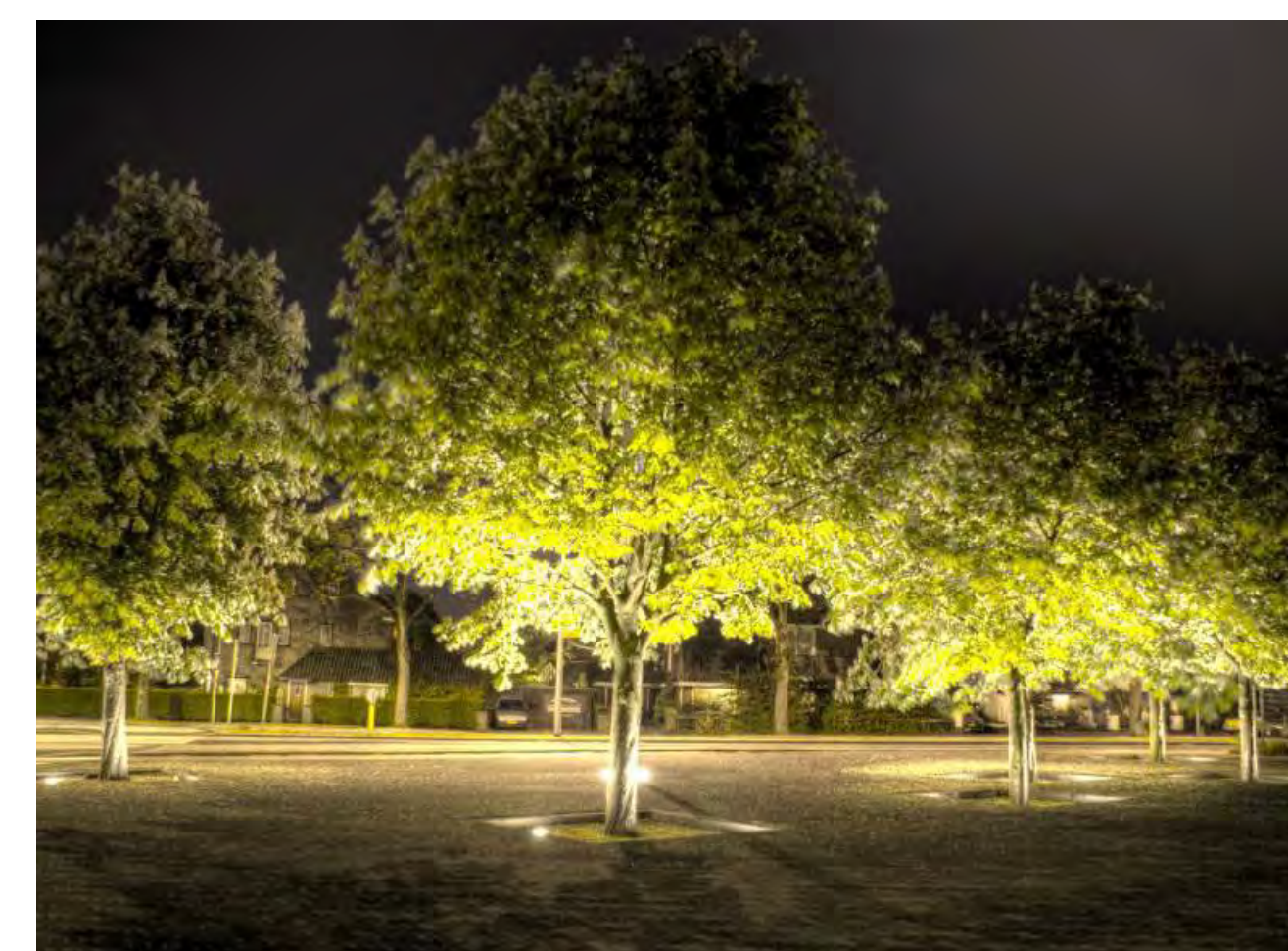
B Stake mounted LED Tree Uplights in raised planters
