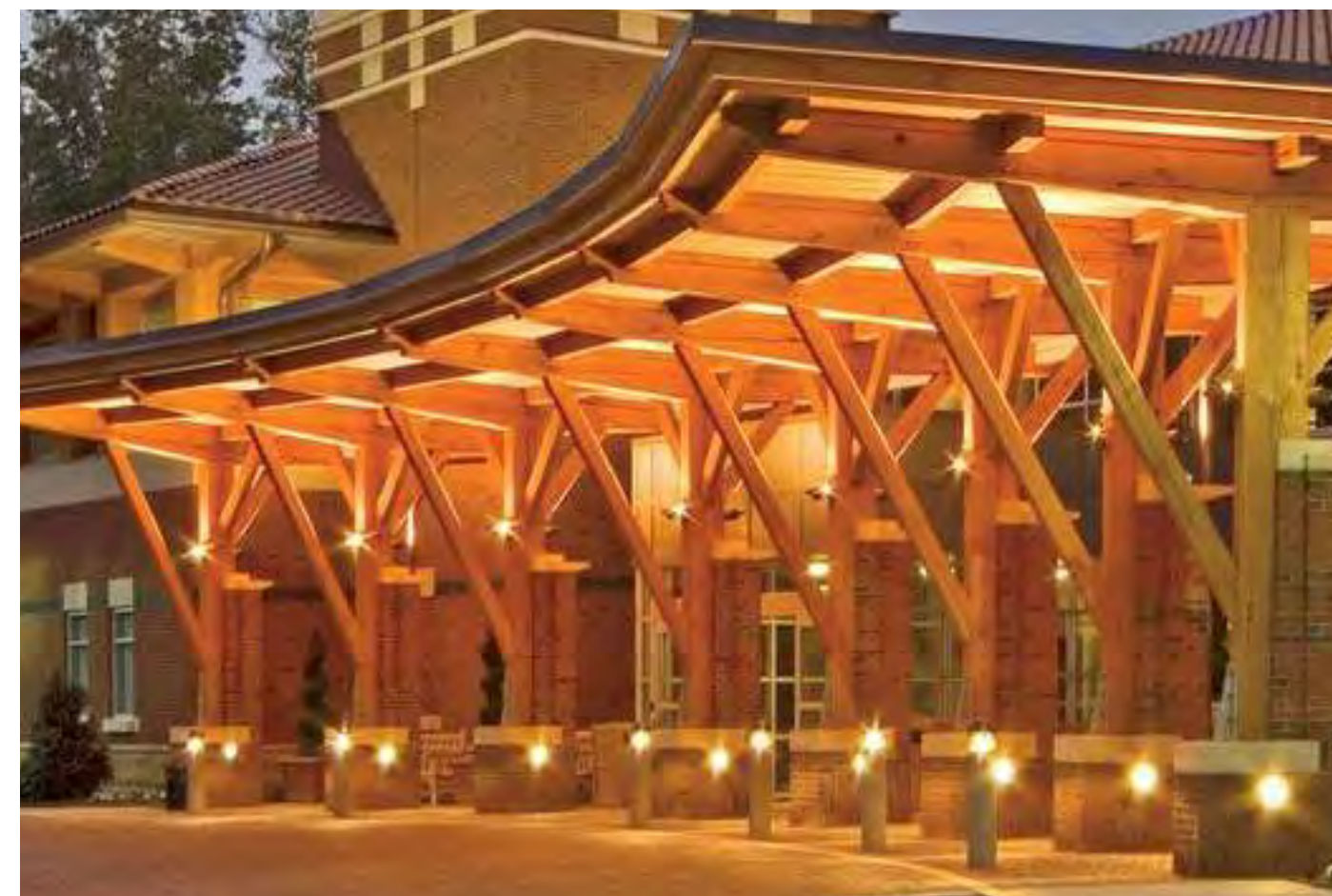
B Column mounted uplights highlight the Heavy Timber Structure above as well as provide warm ambient lighting to the space below
