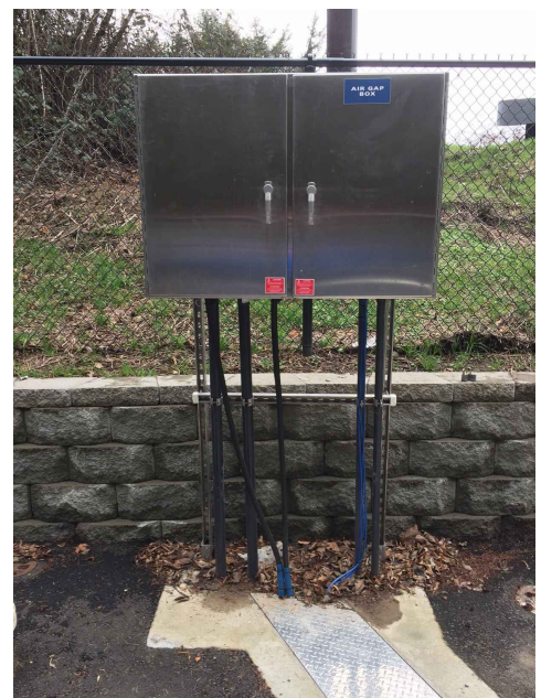
2a DISCONNECT AIR-GAP BOX NTS
