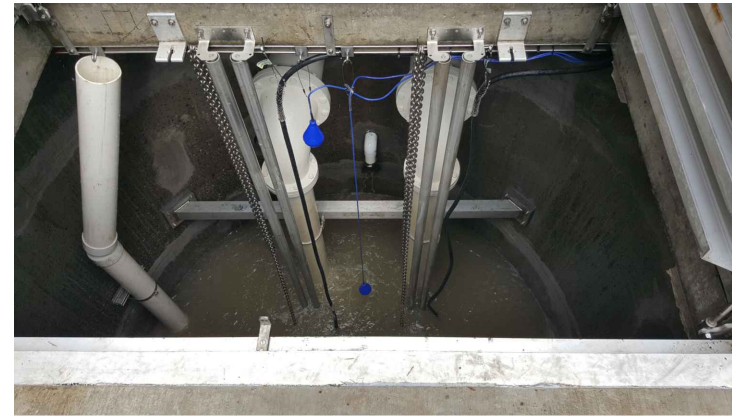
7 CABLE HANGER PHOTO SCALE: NONE
