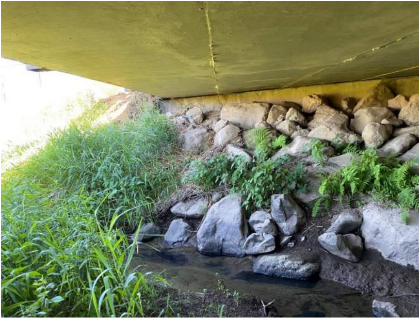
Photo 6 Underside of bridge (looking toward east abutment).
