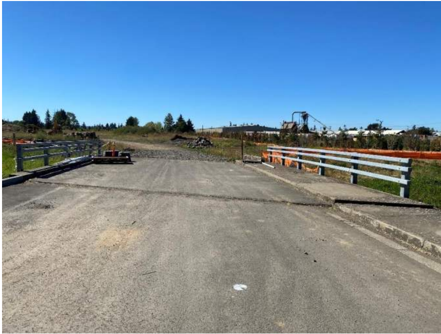
Photo 2 Bridge, looking west.
