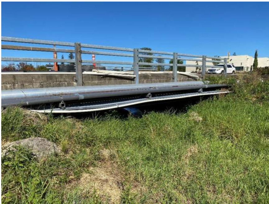
Photo 3 South side of bridge.
