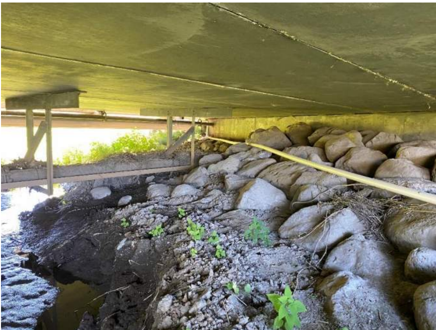
Photo 7 Underside of bridge (looking toward west abutment).
