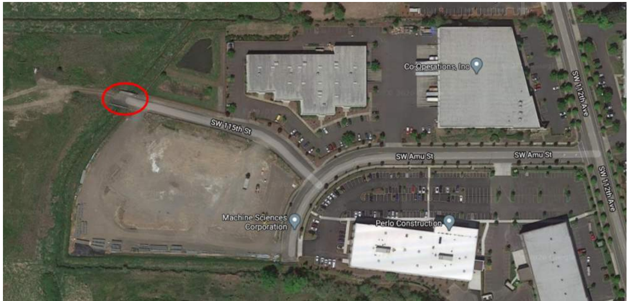
Figure 1 – Aerial of Bridge Location
