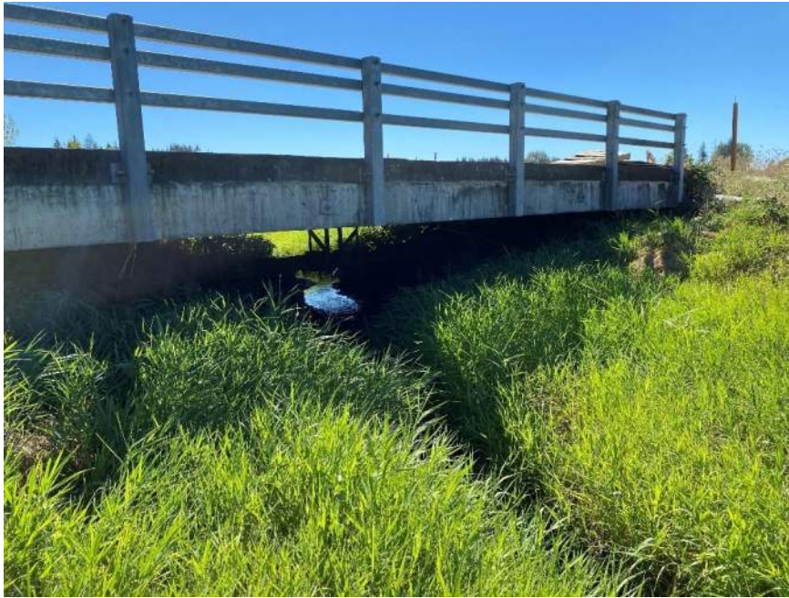
Photo 4 North side of bridge.
