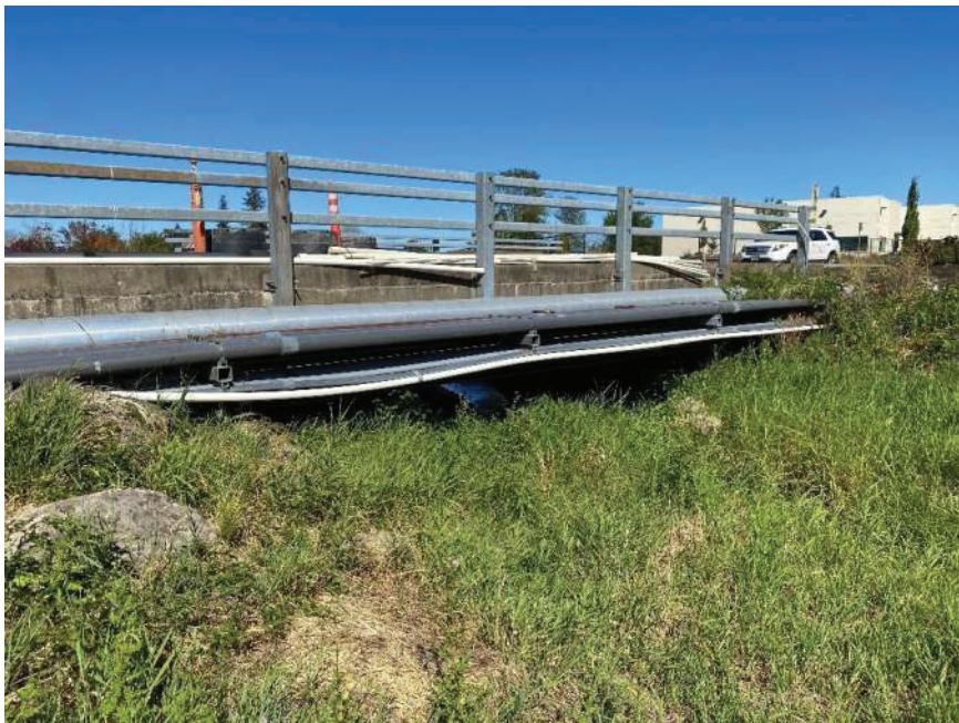
Photo 3 South side of bridge.
