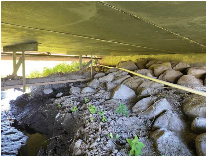
Photo 7 Underside of bridge (looking toward west abutment).
