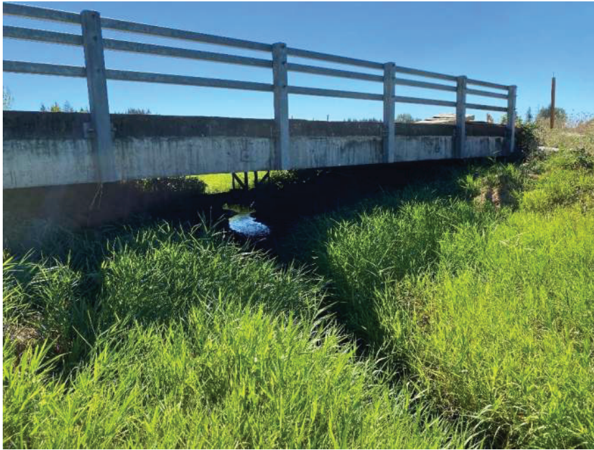
Photo 4 North side of bridge.
