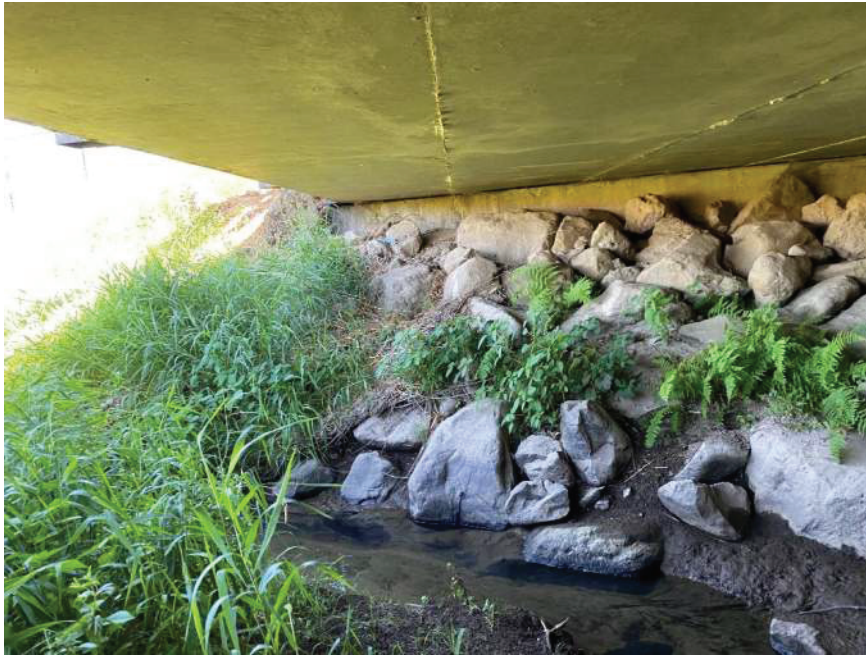
Photo 6 Underside of bridge (looking toward east abutment).
