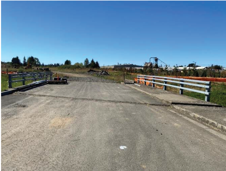
Photo 2 Bridge, looking west.
