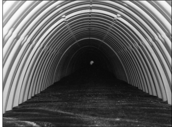
Looking down the Isolator Row
