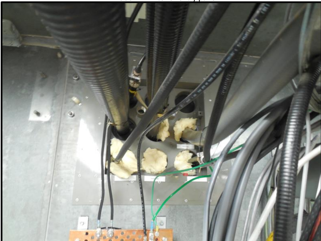
MT SCOTT – Interior entry panel
