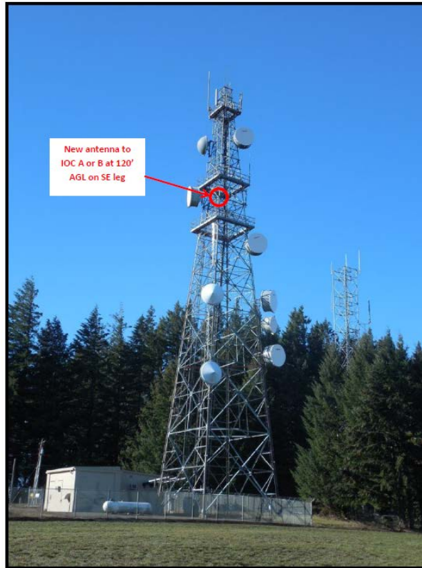
BALD PEAK – Tower view
