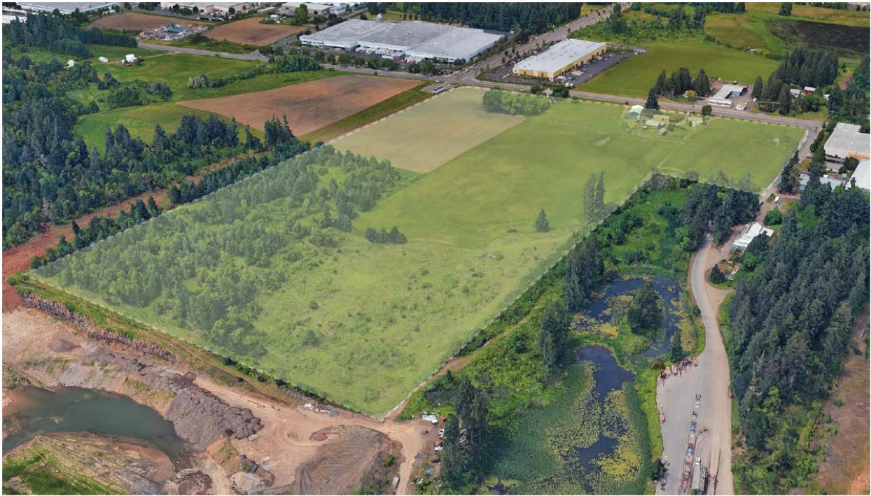
Figure 2. Oblique view of site, looking northwest.
