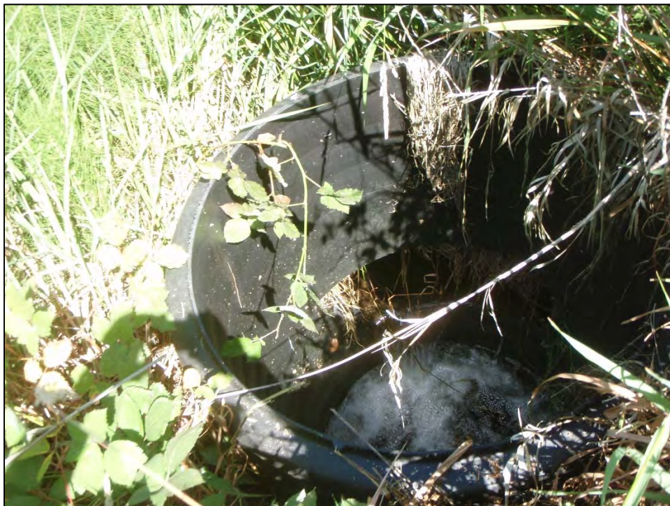
Photopoint 20. Off-site pipe with flowing water.
