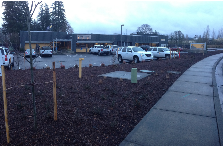
Looking toward existing office building and warehouse from NW corner of site.
