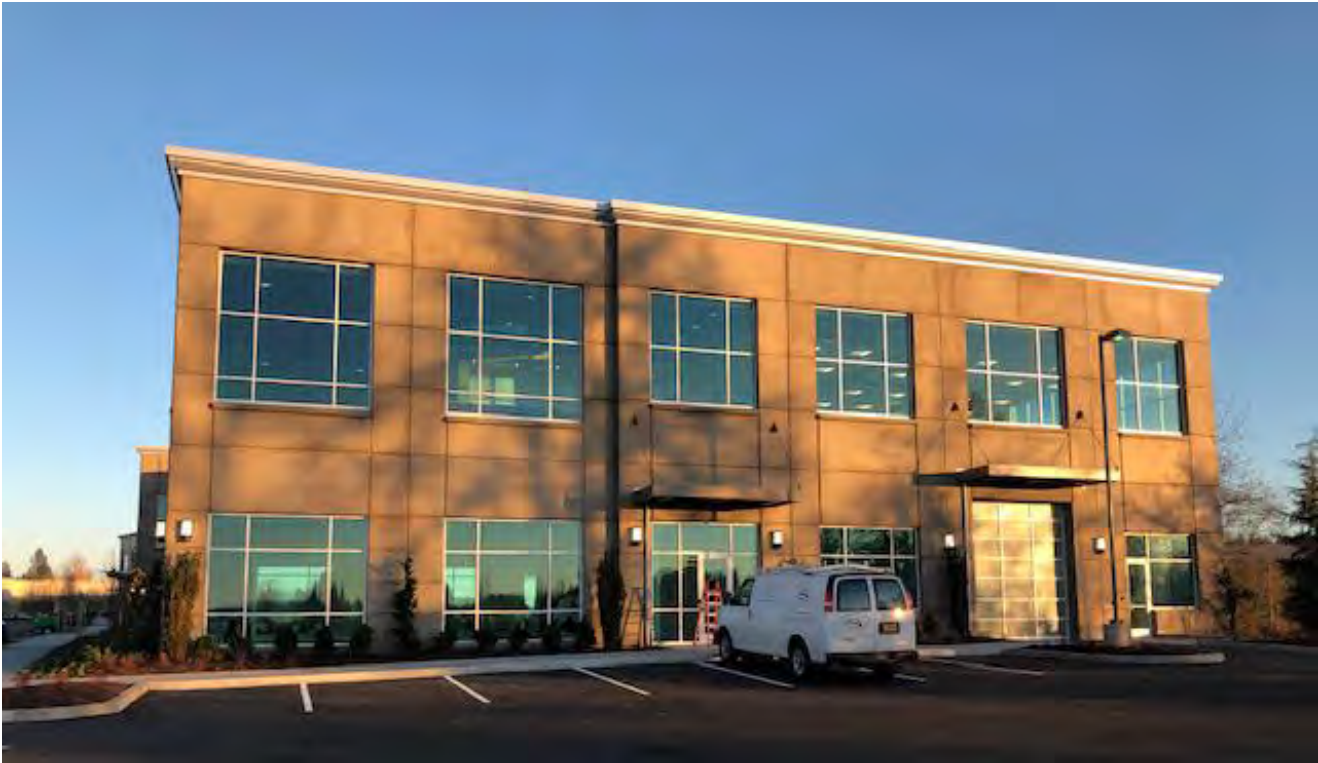
The west side of Hedges B as seen from the Hedges C lot. Hedges B is nearing completion and will be occupied by Perlo Construction. Landscaping is just being installed. The stained precast concrete is seen in the evening yellowing sun 12/6/18.
