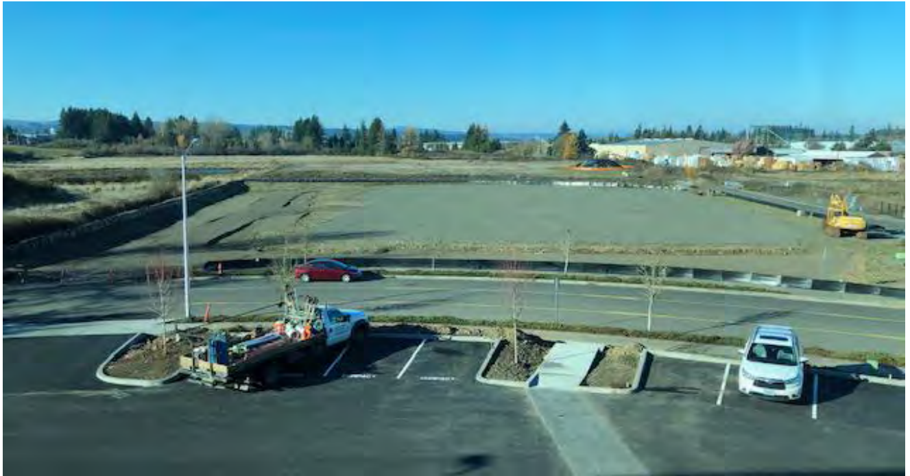
Hedges C as viewed on 12/6/16 from the roof of Hedges B. It shows the site after Early Grading Permit # EC1218-1373 work is complete. This prepared the site for winter weather and for 2019 construction with a new building permit.
