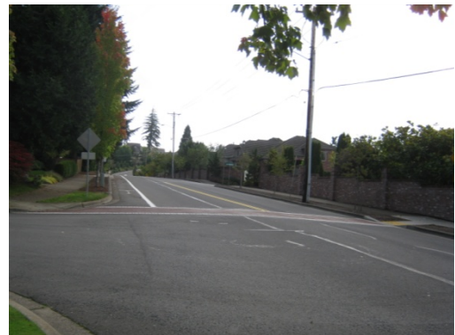
Unsignalized crosswalk on SW 108th Avenue
