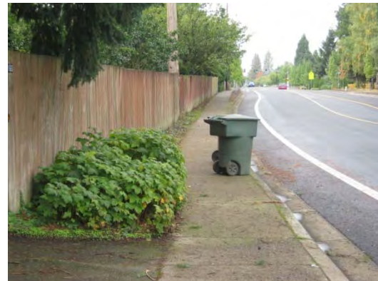
Narrow sidewalk blocked by trash can – Boones Ferry Road
