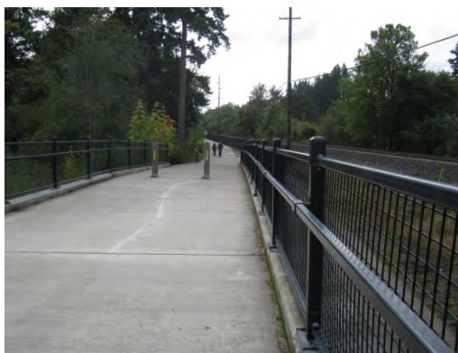
Concrete path in Tualatin Community Park
