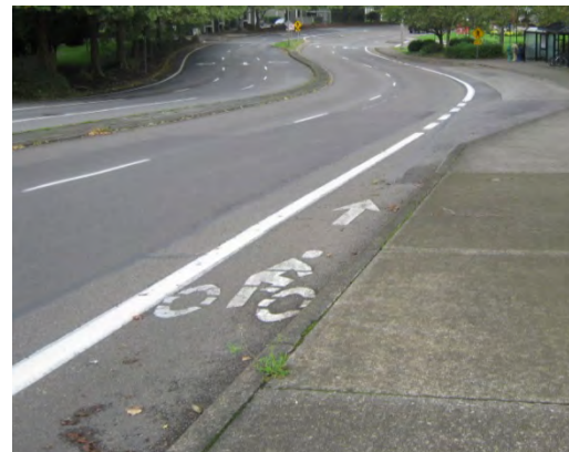
Example of a bike lane on SW Martinazzi Avenue
