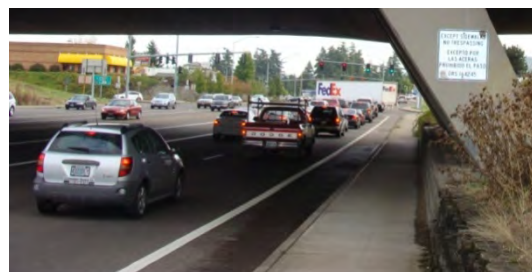
Narrow bike lanes in constrained areas at SW Lower Boones Ferry Road interchange
