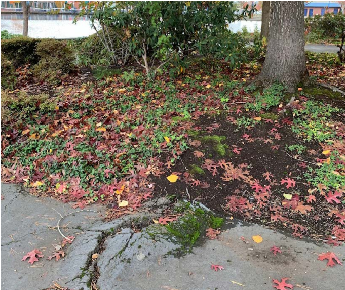
HEAVING / CRACKING PAVING
