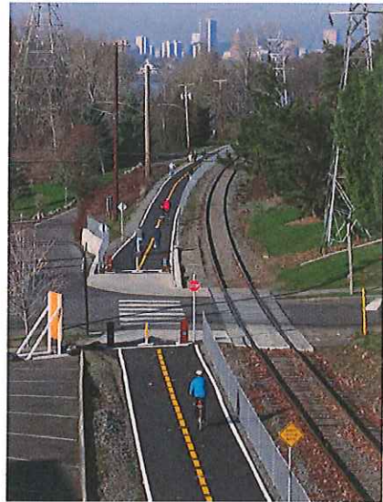
Photo of chain link fence used along a rail-with-trail within a constrained corridor (Springwater Trail).
