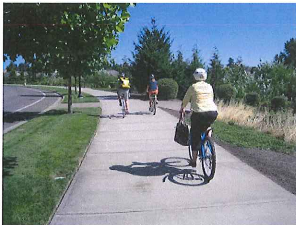
Built section of the Ice Age Tonquin Trail in Wilsonville's Villebois neighborhood.
