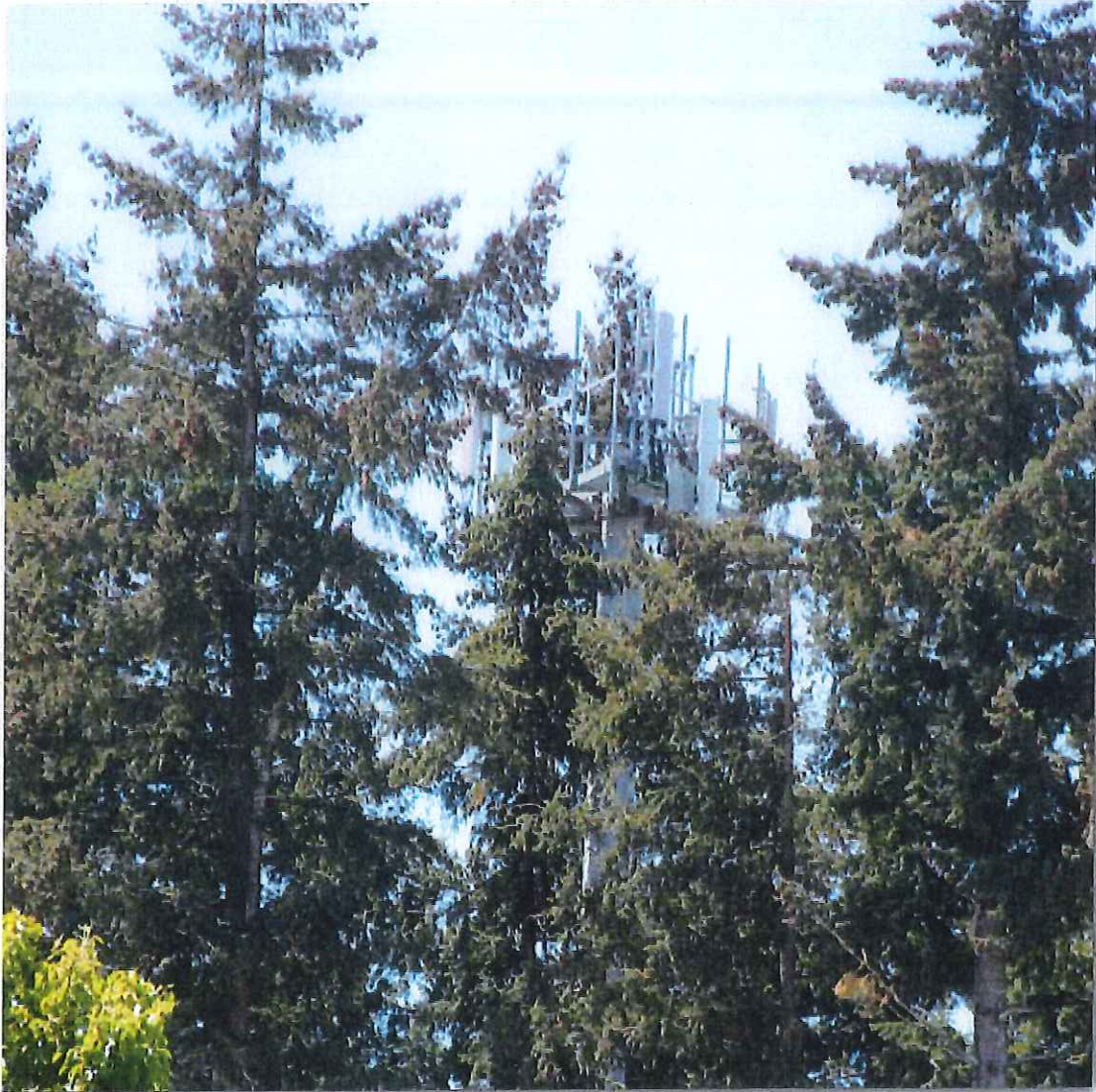
Figure 1: Photo of existing tower surrounded by a dense tree canopy in a near field environment
