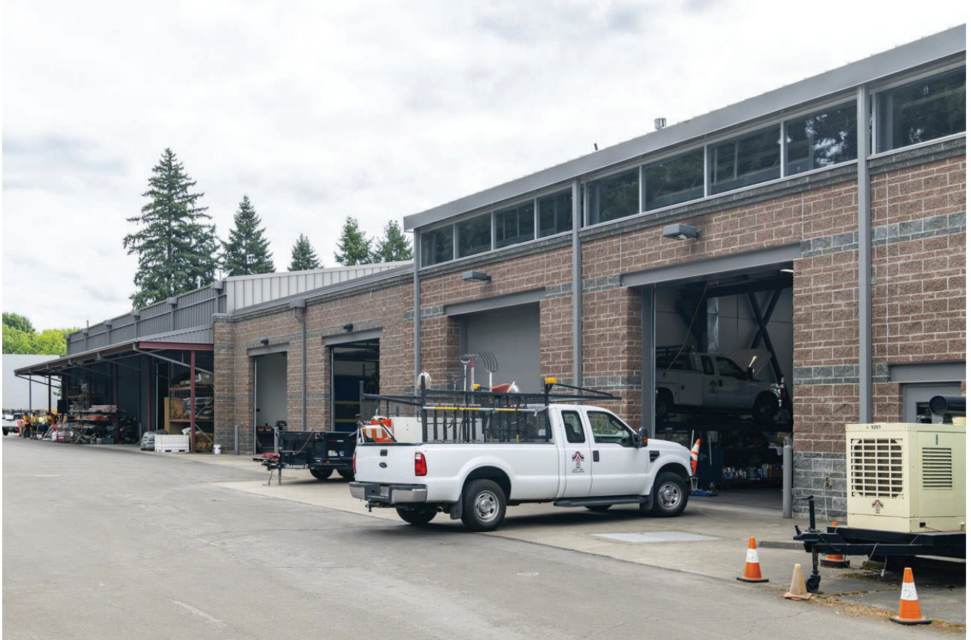
Tualatin City Services Building Warehouse
