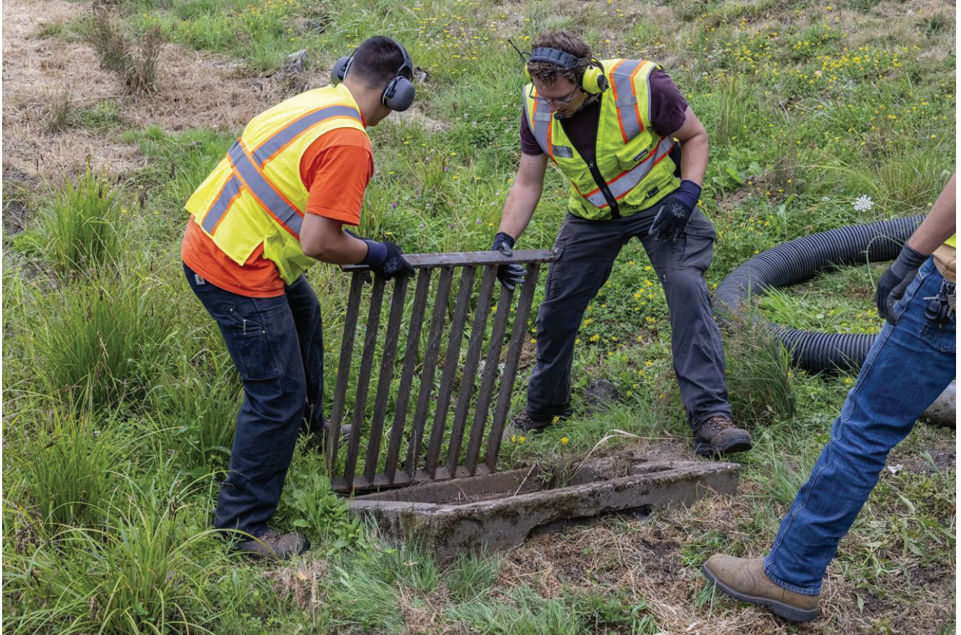
Sewer maintenance work
