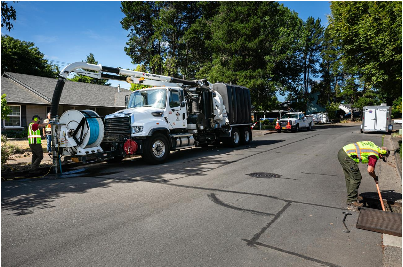
Storm drain cleaning
