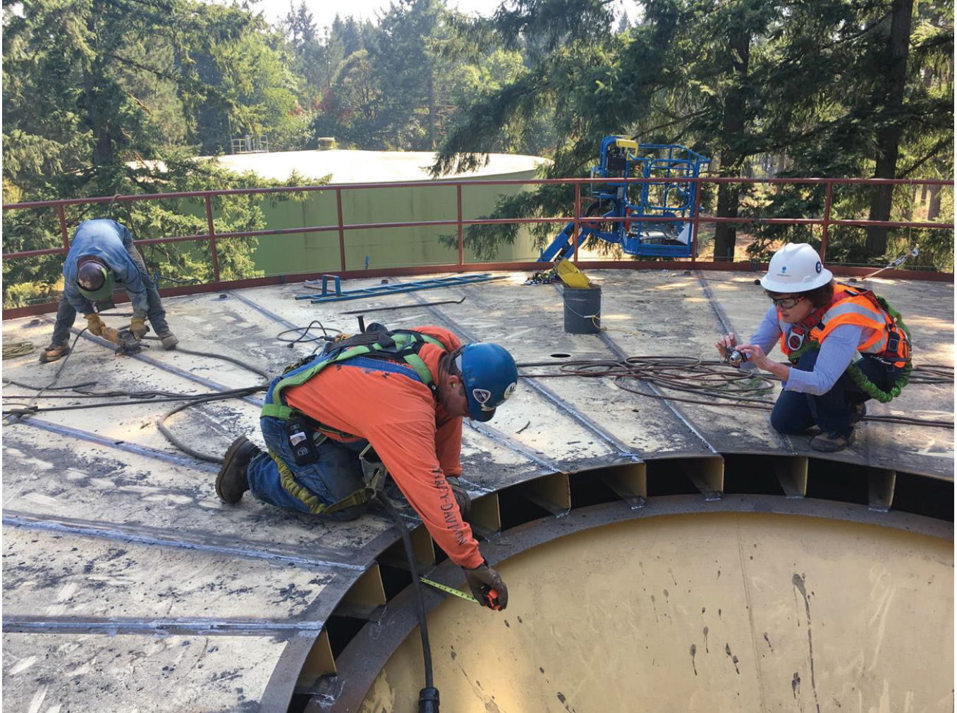
Working on the water reservoirs
