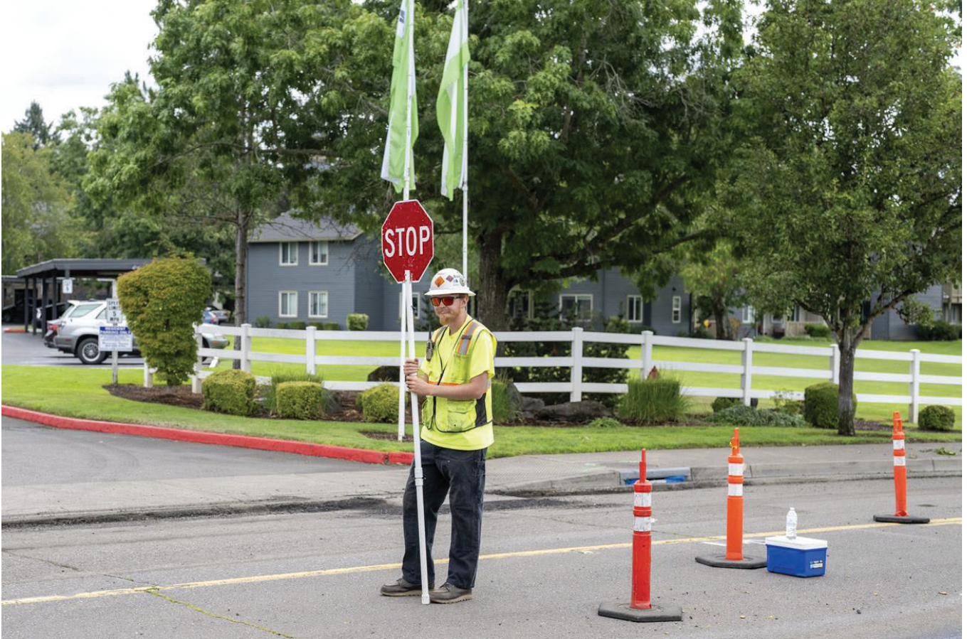
Flagger at road work site
