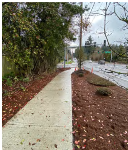
Boones Ferry Road Sidewalk Improvements
