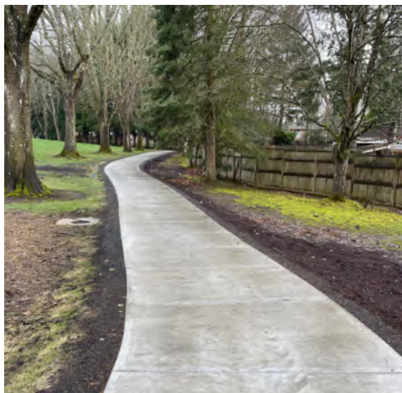
Boones Ferry Road Sidewalk Improvements
