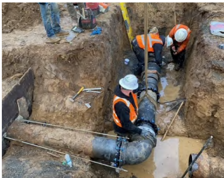
B Level Reservoir Work
