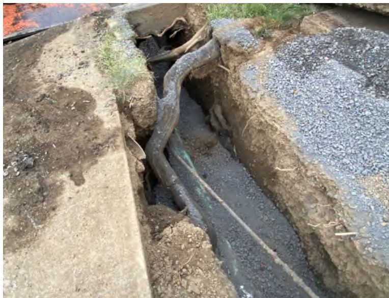
Sewer lateral work - Greenwood
