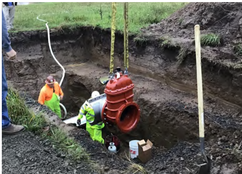
Installing a gate valve
