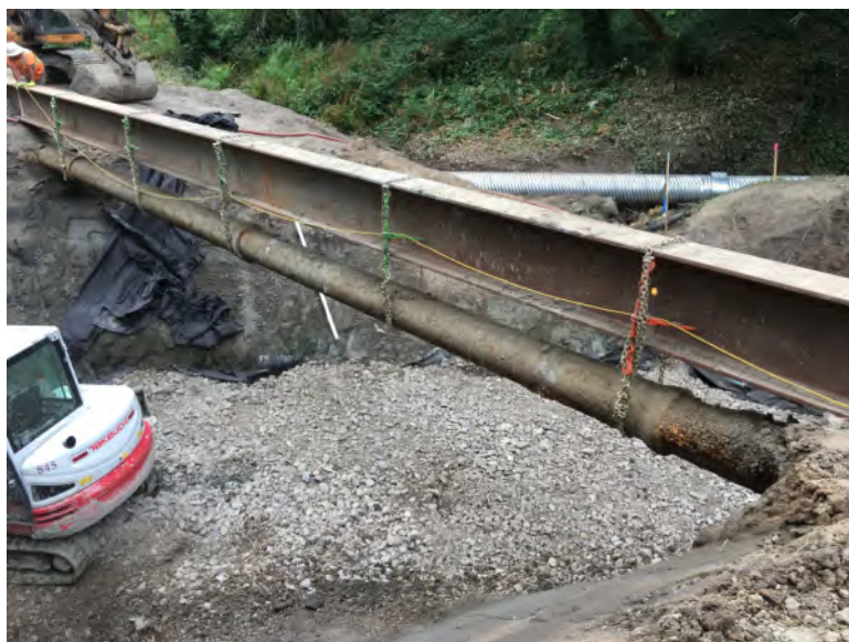
Suspended sewer pipe across creek at Garden Corner curves
