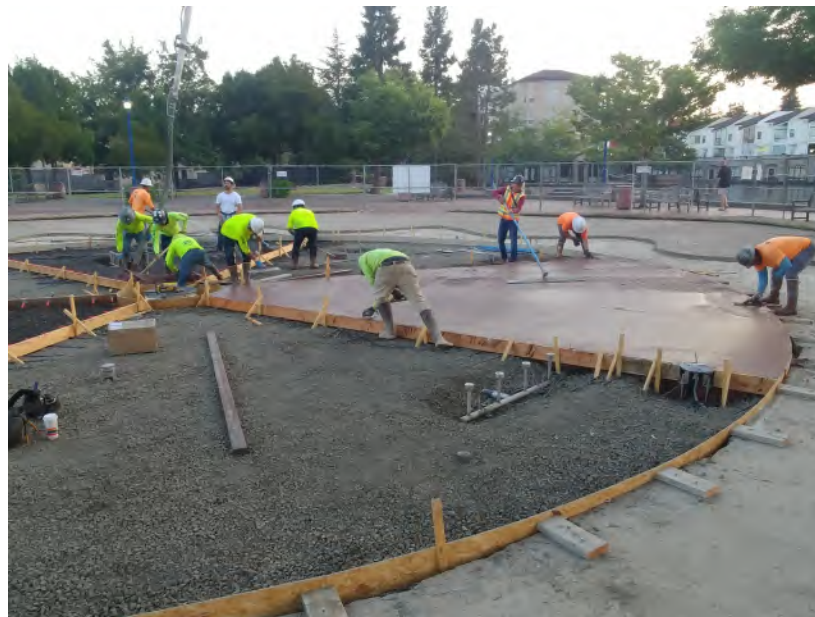
Splash Pad Renovation
