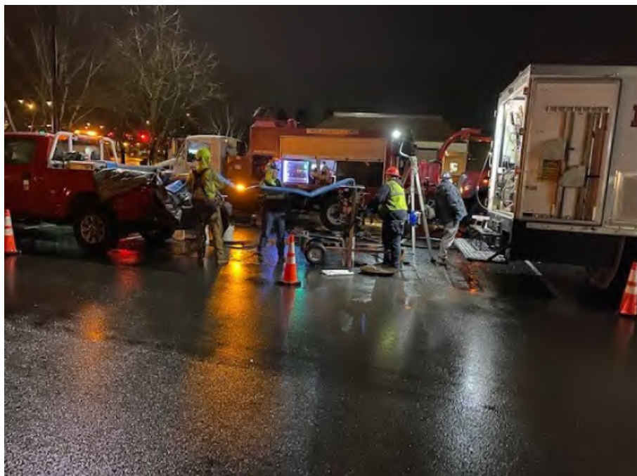
Sewer Main Line Repair
