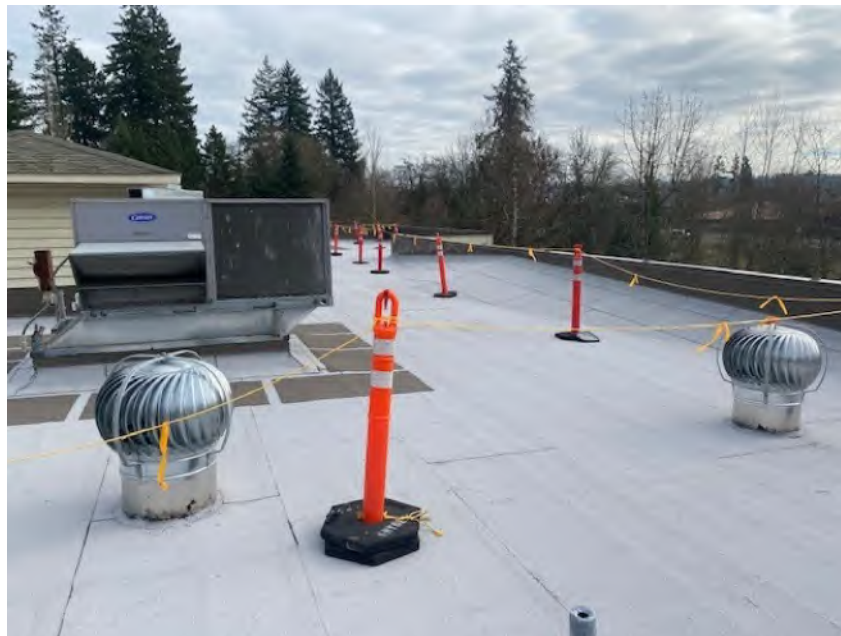
Juanita Pohl Center Roof Project
