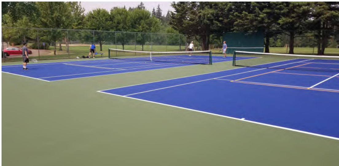
Ibach Tennis Courts Resurfacing
