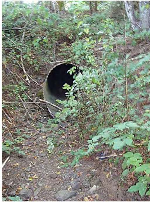
Site location: Culvert at SW Alsea Ct. Photo number: H3-29 Description: Looking downstream, upstream of SW Alsea Ct. Dry channel.
