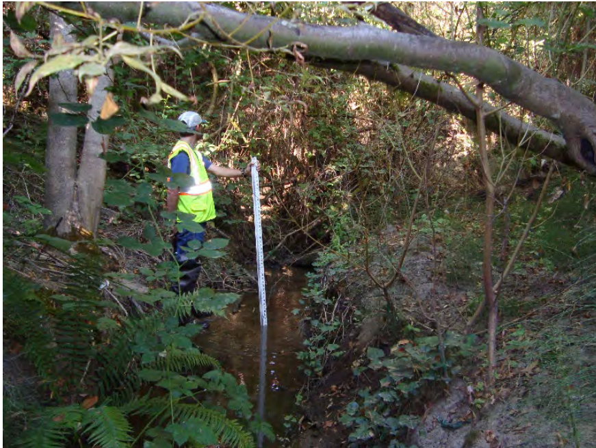
Site location: 300' upstream of confluence with S. tributary Photo number: H3-24 Description: Looking upstream, hard silt in channel, incised
