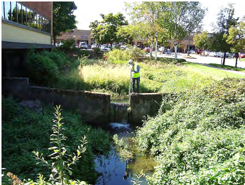
Site location: Upstream of SW Martinazzi Ave. by Shari's restaurant Photo number: N3-2 Description: Nyberg Creek, concrete dam with notch
