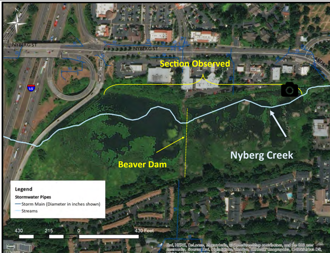
Aerial view of Nyberg Creek Reach #2 (65th Avenue to I-5)
