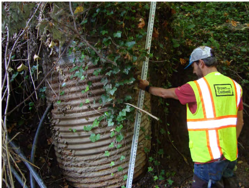
Site location: ~400' upstream from Tualatin River Photo number: S1-4 Description: Corrugated steel pipe (former water intake?) on left bank
