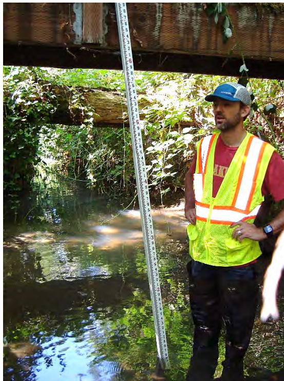
Site location: ~1,200' downstream from SW Borland Rd. Photo number: S1-16 Description: Pedestrian bridge looking downstream, large tree down across channel in distance
