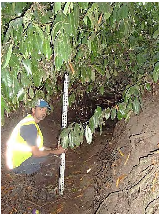
Site location: 200' upstream of SW Alsea Ct. Photo number: H3-30 Description: Looking upstream, narrow defined channel, dry
