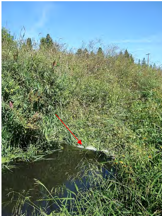
Site location: 400' upstream of SW Nyberg Lane Photo number: N1-6 Description: Looking downstream at top of beaver dam. Red arrow points to top of dam. Drop is approximately 3 feet.
