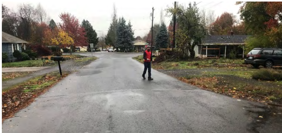
Image 1. Roadside ditches and unimproved roadway at the north end of 93 rd Avenue
