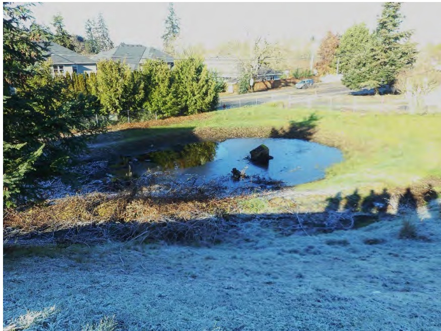
Image 1. Waterford water quality facility as seen from Palouse Lane
