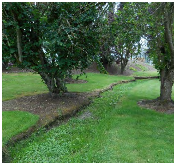
Image 1. Incision and sloughing in the open channel
