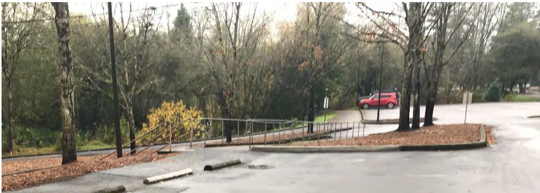
Image 1. Proposed location for water quality facility #1
