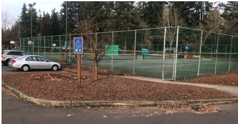
Image 1. Proposed location for Water Quality Facility #1
