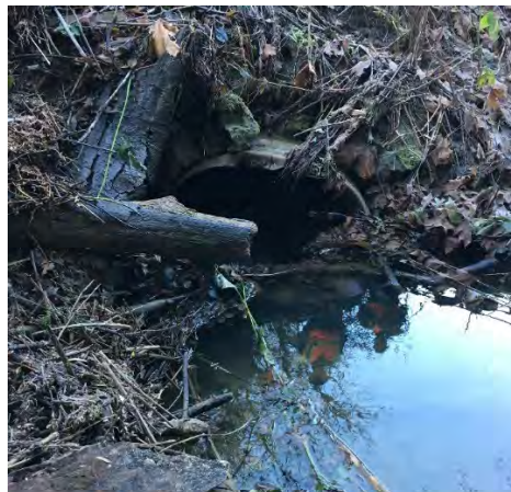
Image 2. Upstream end of culvert
