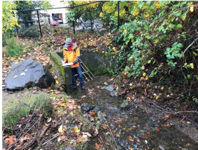
Image 1. Ditch inlet at downstream end of railroad open channel
