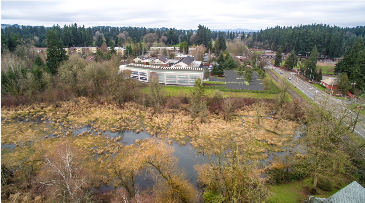
Figure 3 A two-story Civic Center next to the Tualatin Police Department would meet the City's space needs out to 2025.
