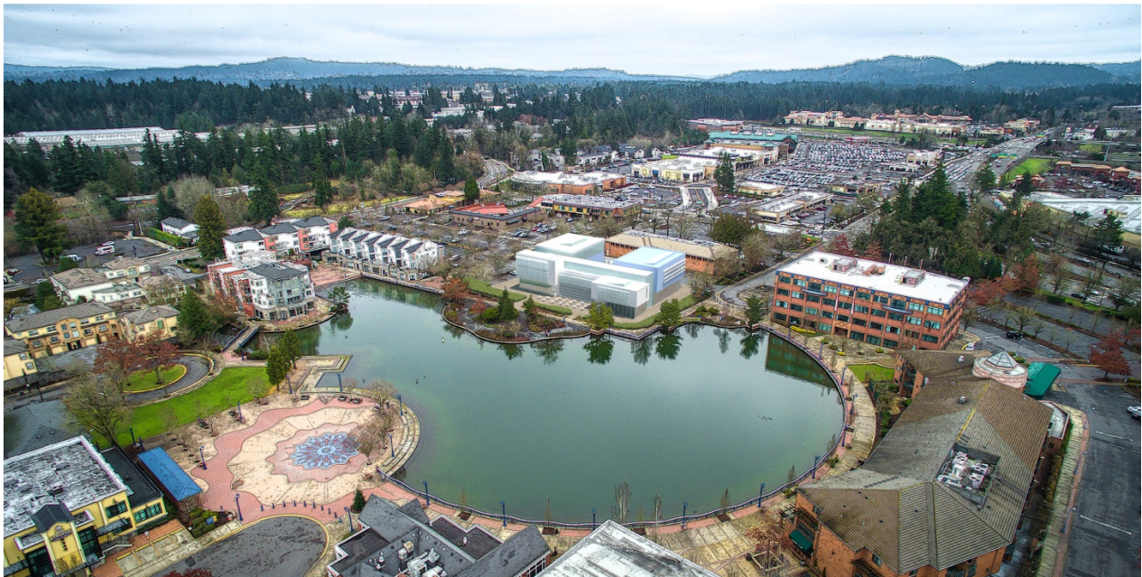
Figure 2 A three-story Civic Center on the Tualatin Commons would meet the City's space needs and would provide additional retail and office space..
