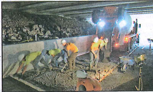
Brown Contracting employees place concrete for path under I-5. Fencing, railing, and daytime lighting will be installed before the trail opens in the Winter of 2015/2016.
