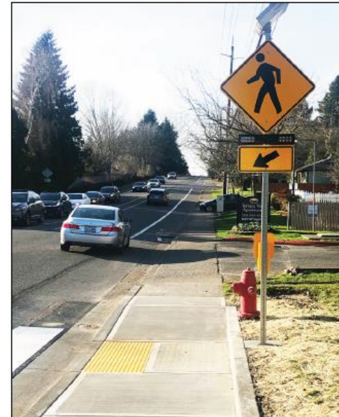
Pedestrian-activated signal at crosswalk, SW Sagert St and SW Wampanoag Dr
