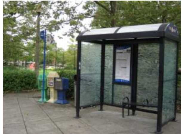
Bus stop for TriMet line Nos. 76 and 96
