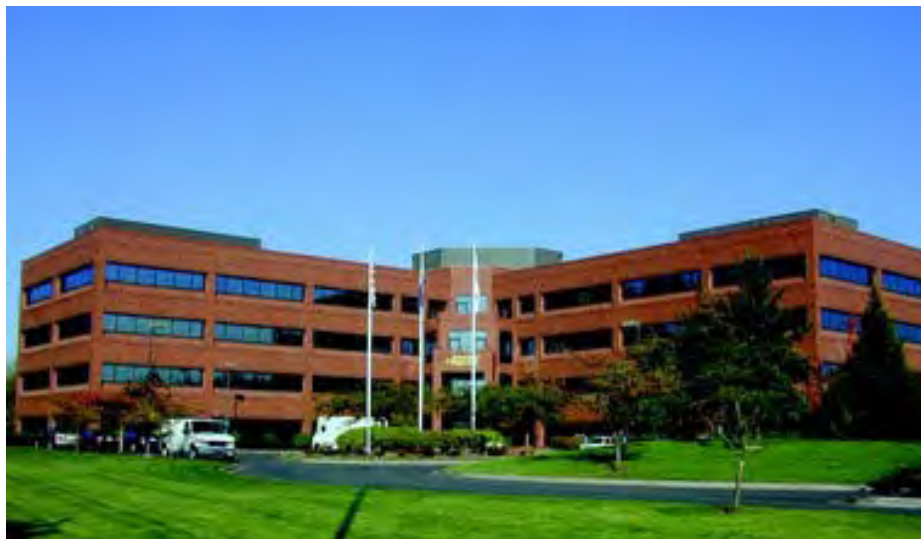
Figure 30 Mentor Graphics Headquarters Office Building in Wilsonville.
