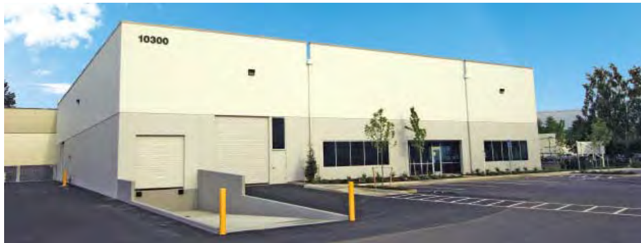
Figure 29 Example of typical flex industrial building, located in Tualatin.
