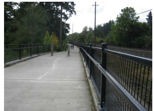
Concrete path in Tualatin Community Park
