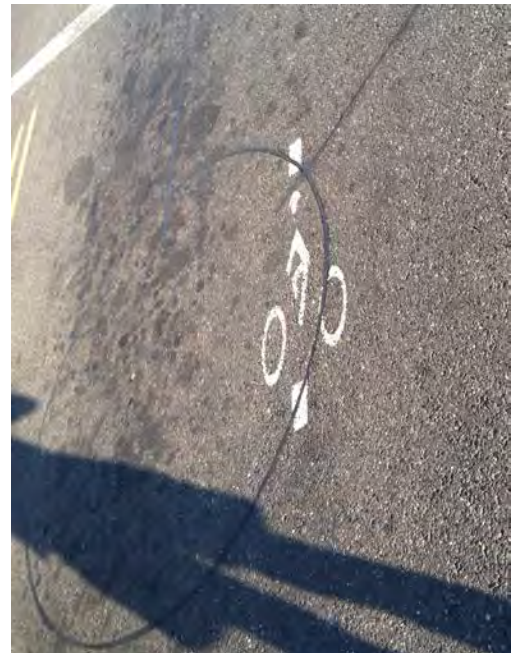
Example of a Bicycle Detector Loop
