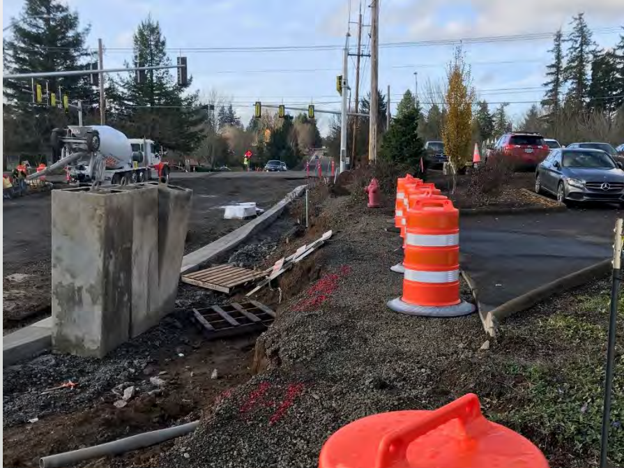
TPC looking west toward SW 65 th Avenue
