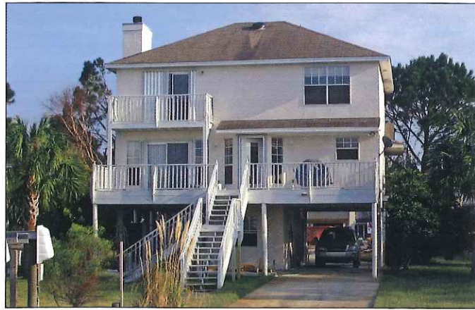
Elevated home on pile foundation
