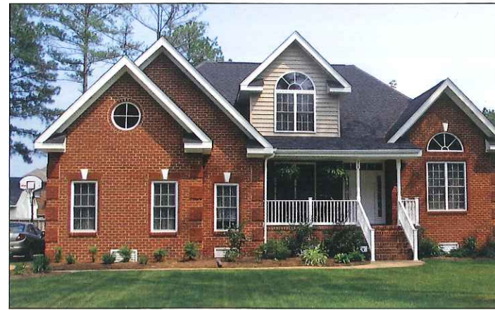
Elevated home on crawl space foundation
