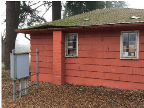
Side Elevation of Garage (north)
