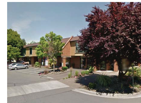
Rear Elevation Detail (west)
