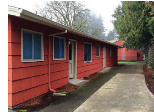
Rear Elevation (north)
