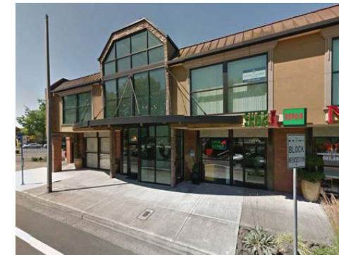
Building Entry (east)
