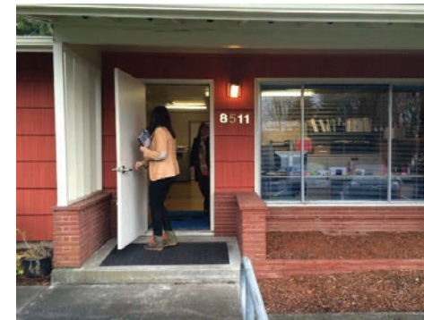
Front Entry (south)
