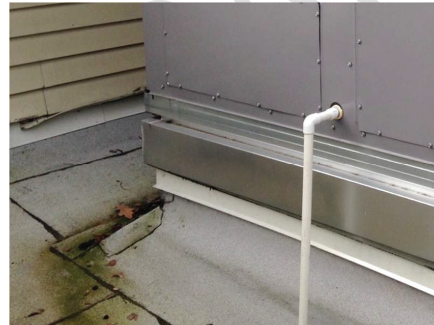
Figure B30.1 Staff photo of roof condition above Activity Room space
