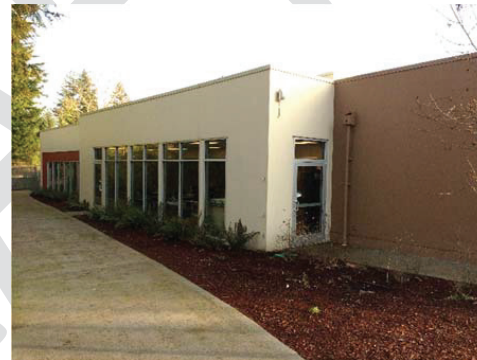
Side Elevation (north)
