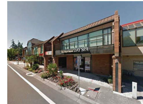
Front of Building (east)
