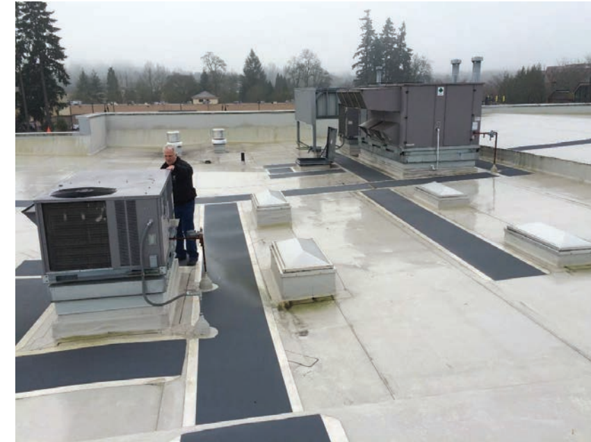
Figure B30.1 Rooftop conditions observed
