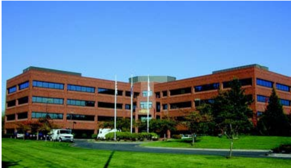
Figure 30 Mentor Graphics Headquarters Office Building in Wilsonville.
