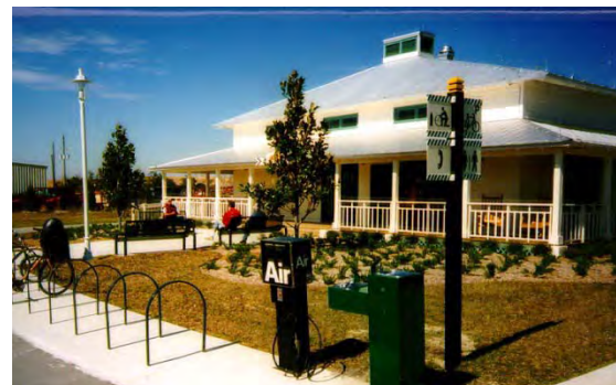
A major trailhead with bike racks, air compressor (for bicycle tires), water fountain, restrooms, phone, and benches.
