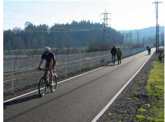
Wildlife friendly fence with 6-inch vertical gap at the bottom for small animal passage (Springwater Trail).
