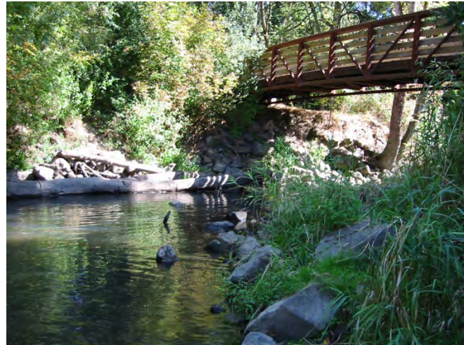
Bridge design allows for wildlife to pass beneath it.
