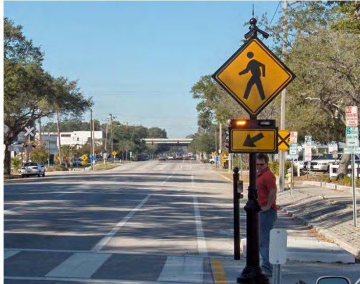
Rectangular rapid flashing beacons at a trail/roadway crossing.
