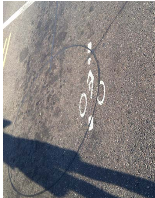
Example of a Bicycle Detector Loop
