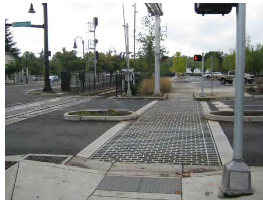
Park and ride entrance crosswalk
