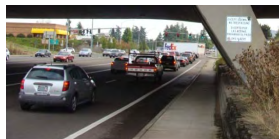
Narrow bike lanes in constrained areas at SW Lower Boones Ferry Road interchange
