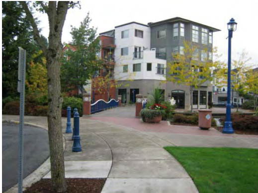
Example of mixed use development in the Town Center area
