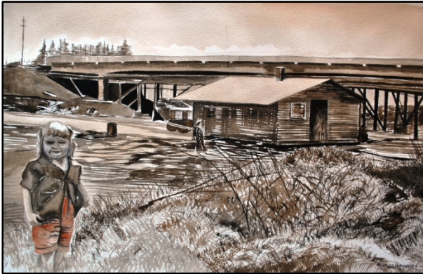
1950 – 1959: Construction of I-5 Freeway
