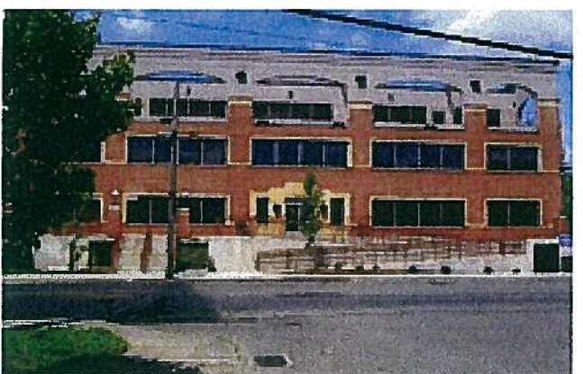
Aspen Place – Boones Ferry Road
