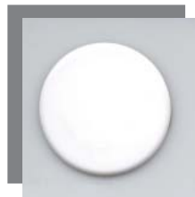
Finished hidden sprinkler head installation.
