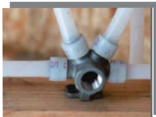
Installation of piping and head manifold during construction
