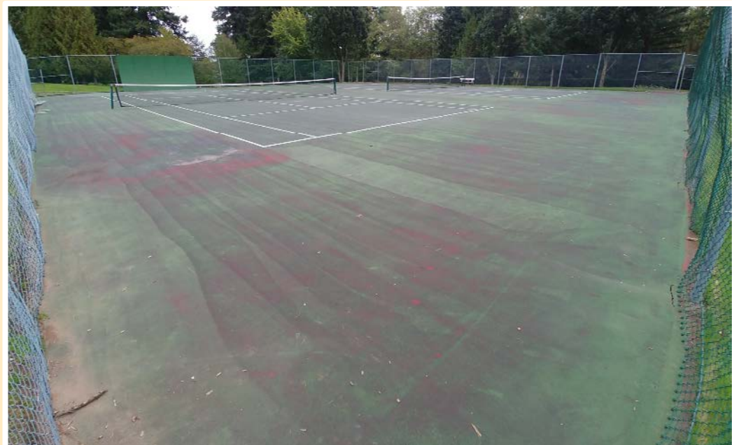
ATFALATI PARK DETERIORATING TENNIS COURT SURFACE
