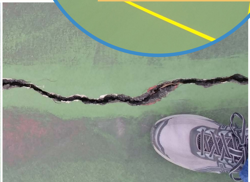
ATFALATI PARK DETERIORATING TENNIS COURT SURFACE
