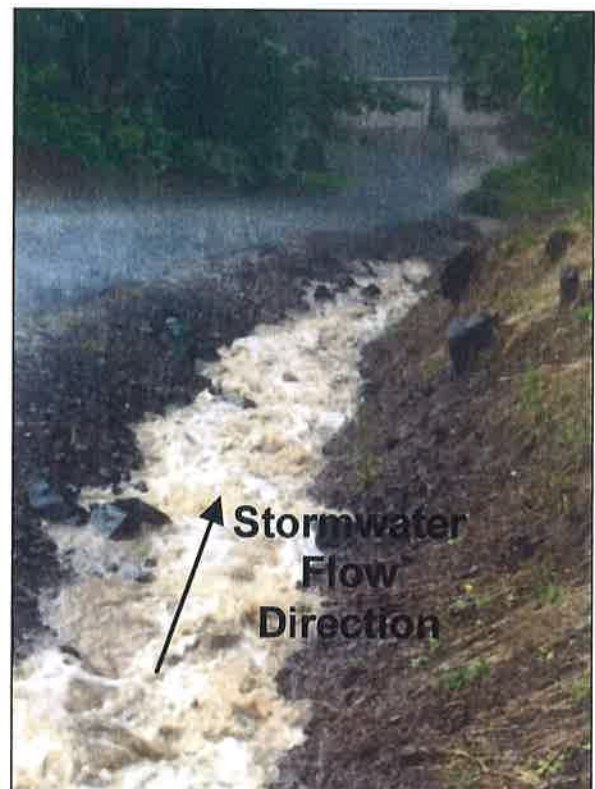
Photo A2. Channel conveying Boones Ferry Road drainage across the Lucini property.
