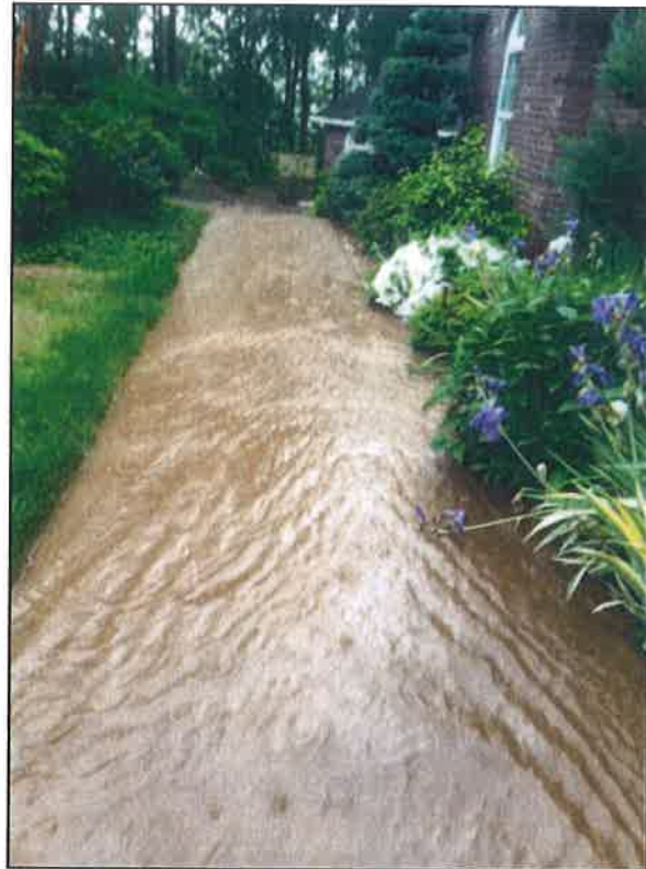
Photo A5. The front lawn drained its flood waters into the walkway and porch in front of the house.
