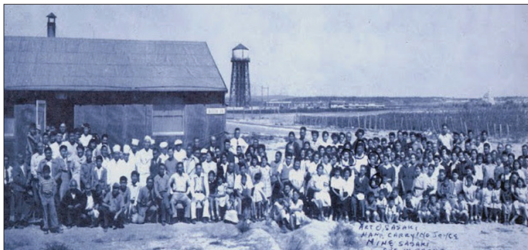
Camp Minidoka Block 39 Barrack 12 in Jerome County, Idaho, in 1943.
