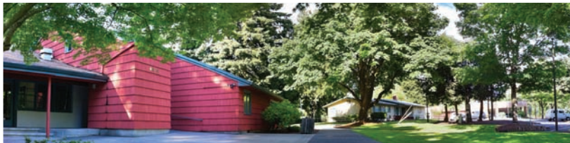
The Van Raden Community Center, Lafky House and Juanita Pohl Center will be used as a multigenerational complex to expand recreation programs.
