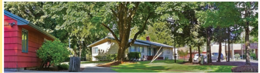
The Van Raden Community Center, Lafky House, and Juanita Pohl Center will be used as a multigenerational complex to expand recreation programs.
